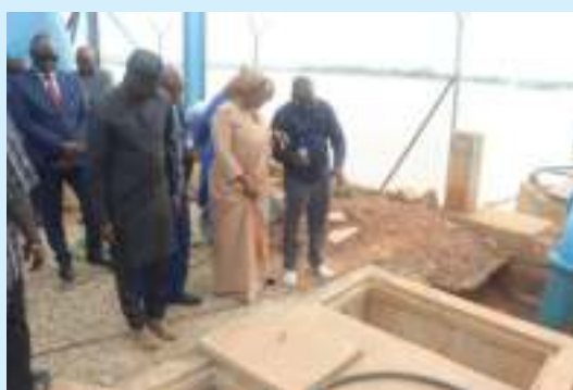
Station de KALABANBOUGOU
